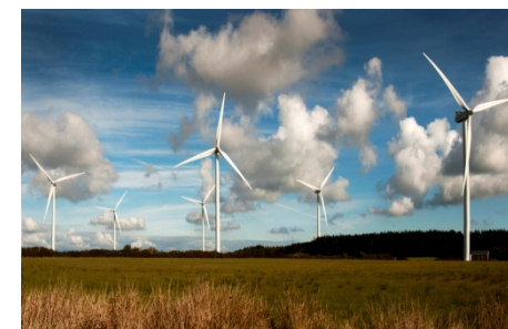
Goonhilly Downs Wind Farm
