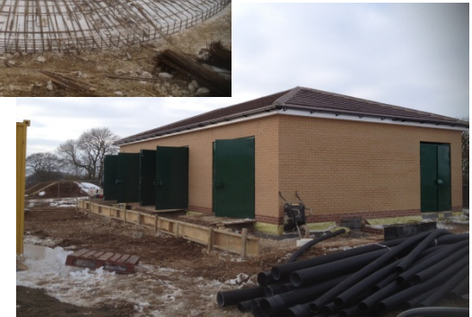
Sancton Hill windfarm under construction
