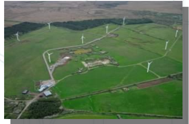
Goonhilly - Construction commenced May, 2010.
