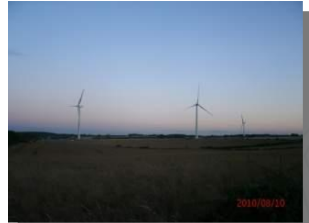
Loscar - Turbines erected August, 2010.
