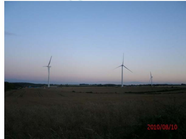
Loscar - Turbines erected August, 2010.
