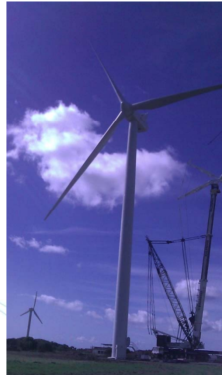
Goonhilly - First turbine erected 28-Aug-10..
