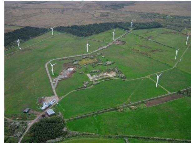
Goonhilly - Construction commenced May, 2010.
